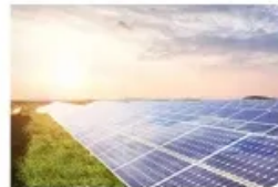
Energy Storage System
